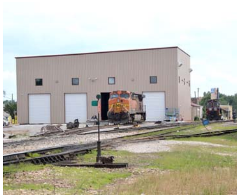
The Arkansas & Missouri Railroad's new $2.5 million locomotive facility.
